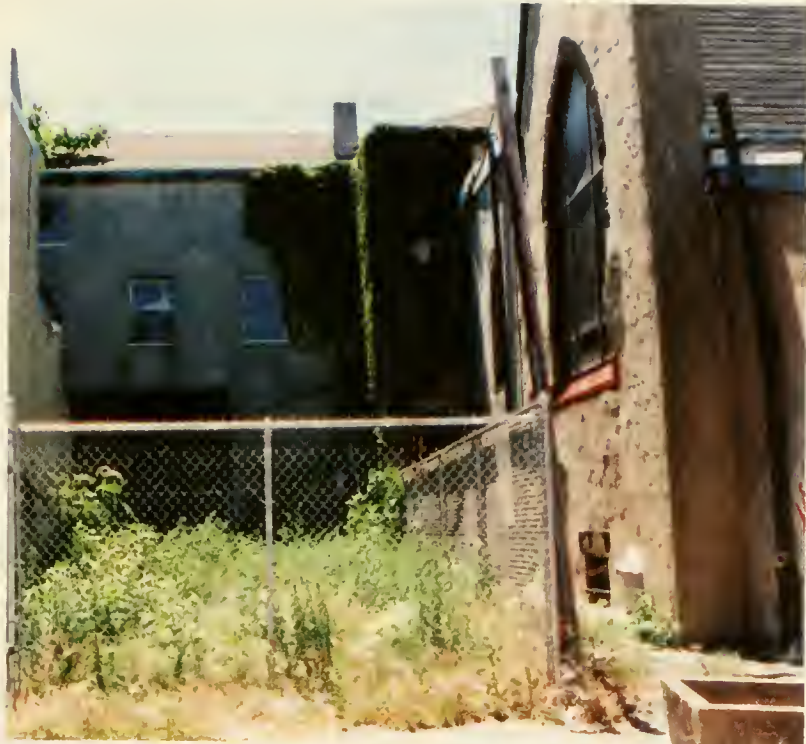
East Elevation of Church Building (R)
